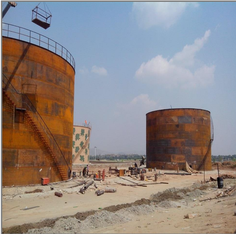
Crude Oil Storage Tanks 20,000 bbls Nashpa Oil Field
